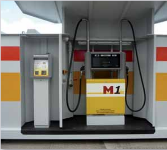
Dispenser recess with filling pump Gilbarco 130 / 40 l/min
