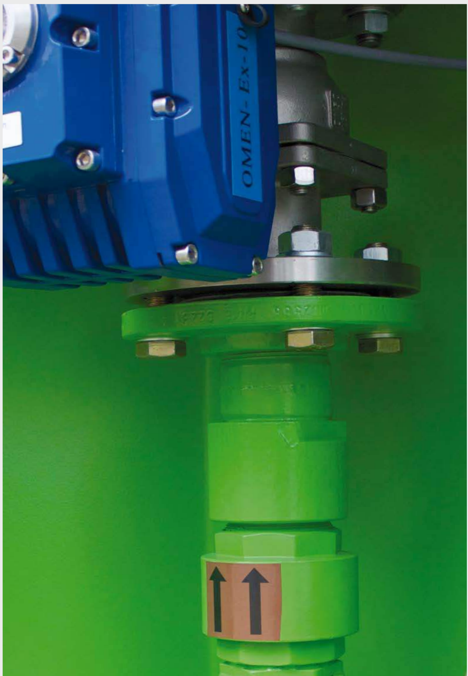
flame arresters in transfer niche
