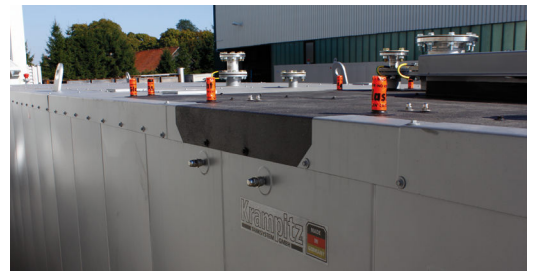
mounting plug for access ladder and railing
