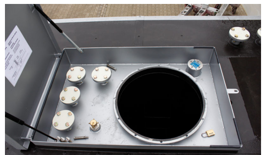
protective cover element, inspection opening and connection interfaces
