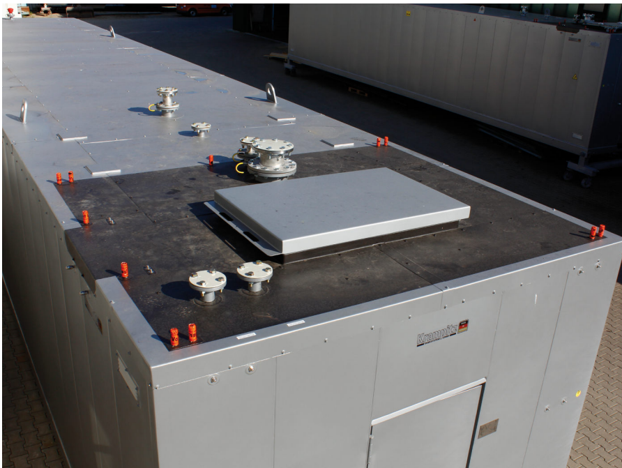
anti-slip coating on accessible roof area
